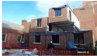
Figure no. 9. Modular building made of prefabricated 3D modules (Smith, 2016)
